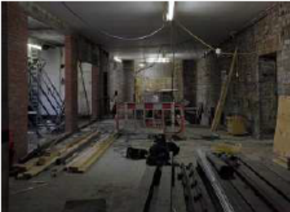
General View: Main Entrance (looking West towards Box Office).
