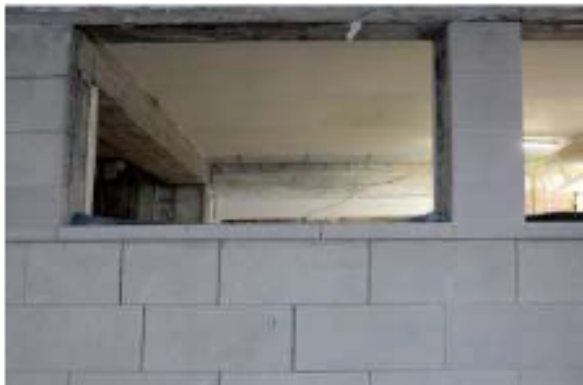
General View: new cast stone to front elevation (Ground Floor).
