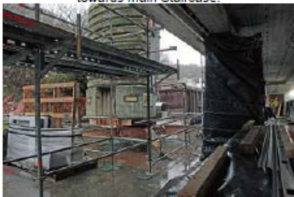
General View: Auditorium West wing (looking North). NB: base of site crane visible.
