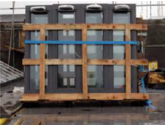
Auditorium Roof Light: patent glazing.
