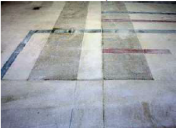
General View: Main Entrance terrazzo flooring exposed.
