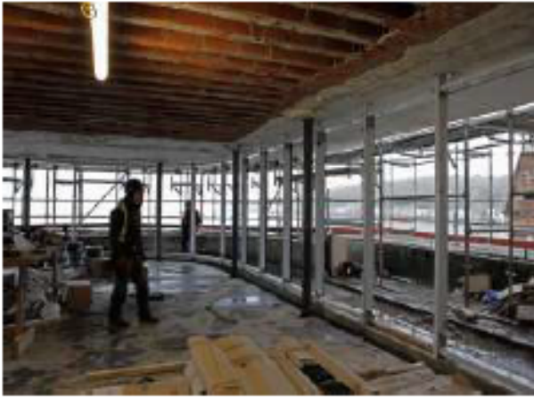
New curtain walling line to the new Exhibition/Function room (towards Argyll St)
