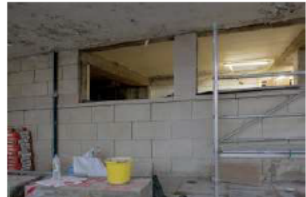
General View: front elevation.
