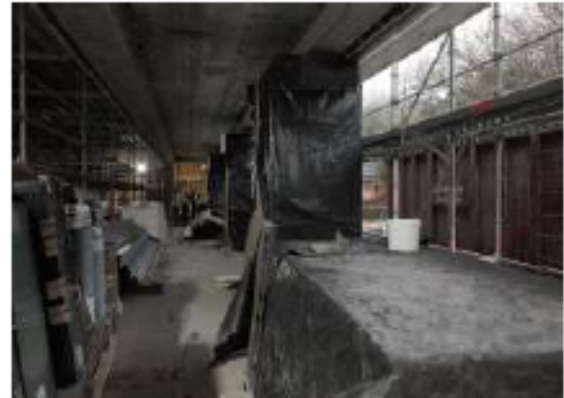
General View: Auditorium West wing (looking south).
