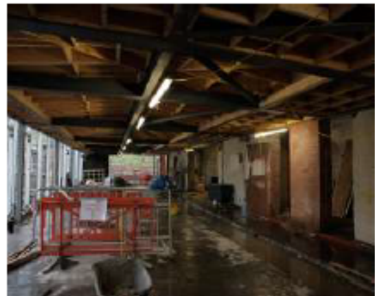
New Offices: General view B (looking West).
