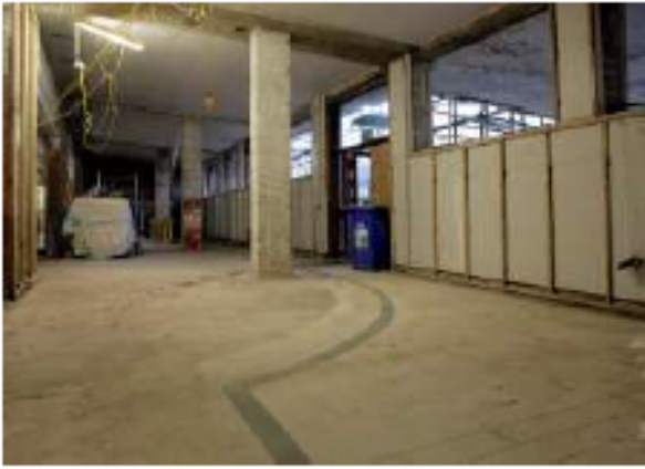
General View: New Exhibition area front wall.
